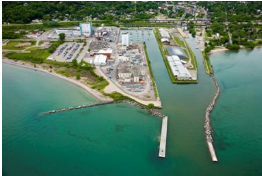
Figure 2 – Site 1, Port Hope Conversion Facility and Centre Pier looking north
