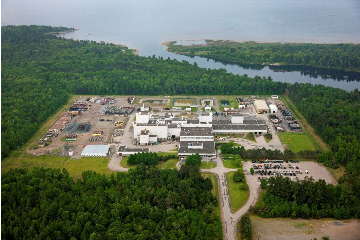
Figure 2 – Aerial View of the Blind River Refinery
