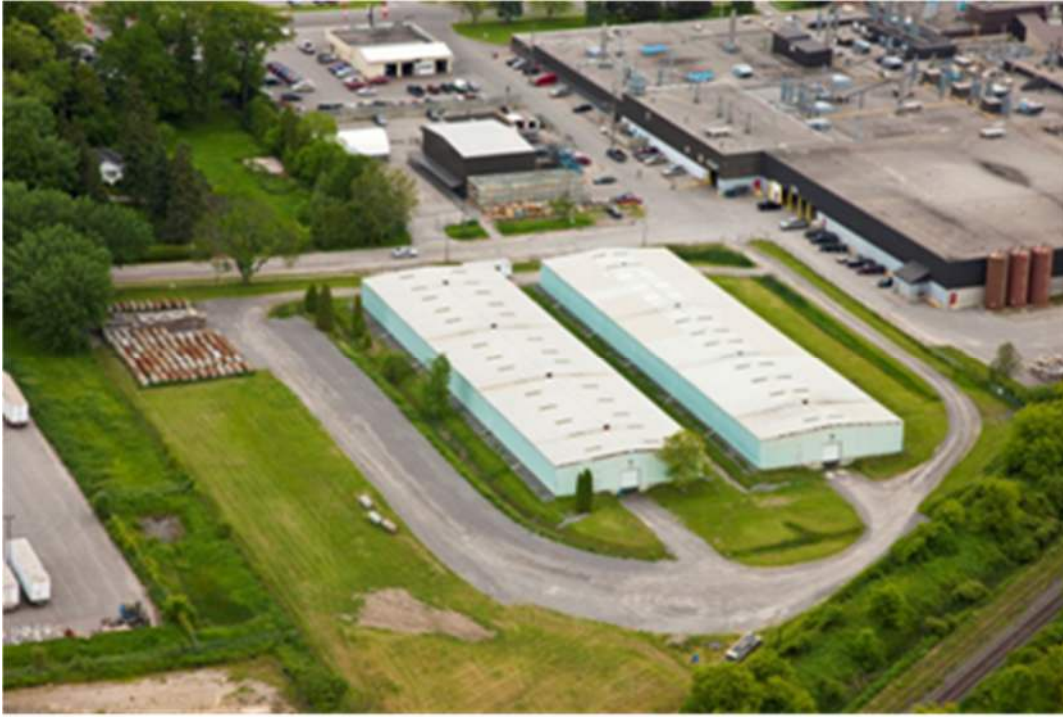
Figure 2 – Site 2 - Storage Facility
