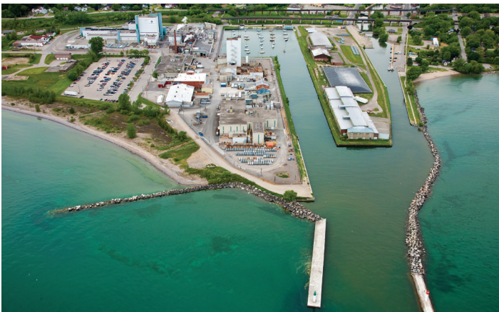
Figure 1 | Port Hope Conversion Facility Main Site and Centre Pier
