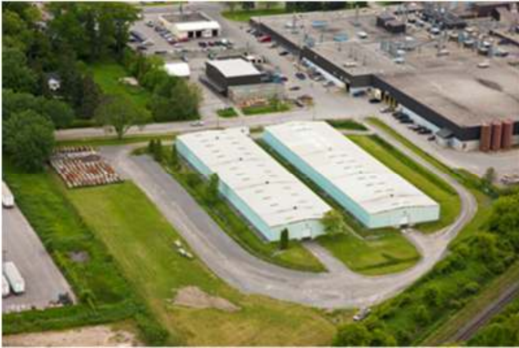
Figure 2 – Site 2 - Storage Facility
