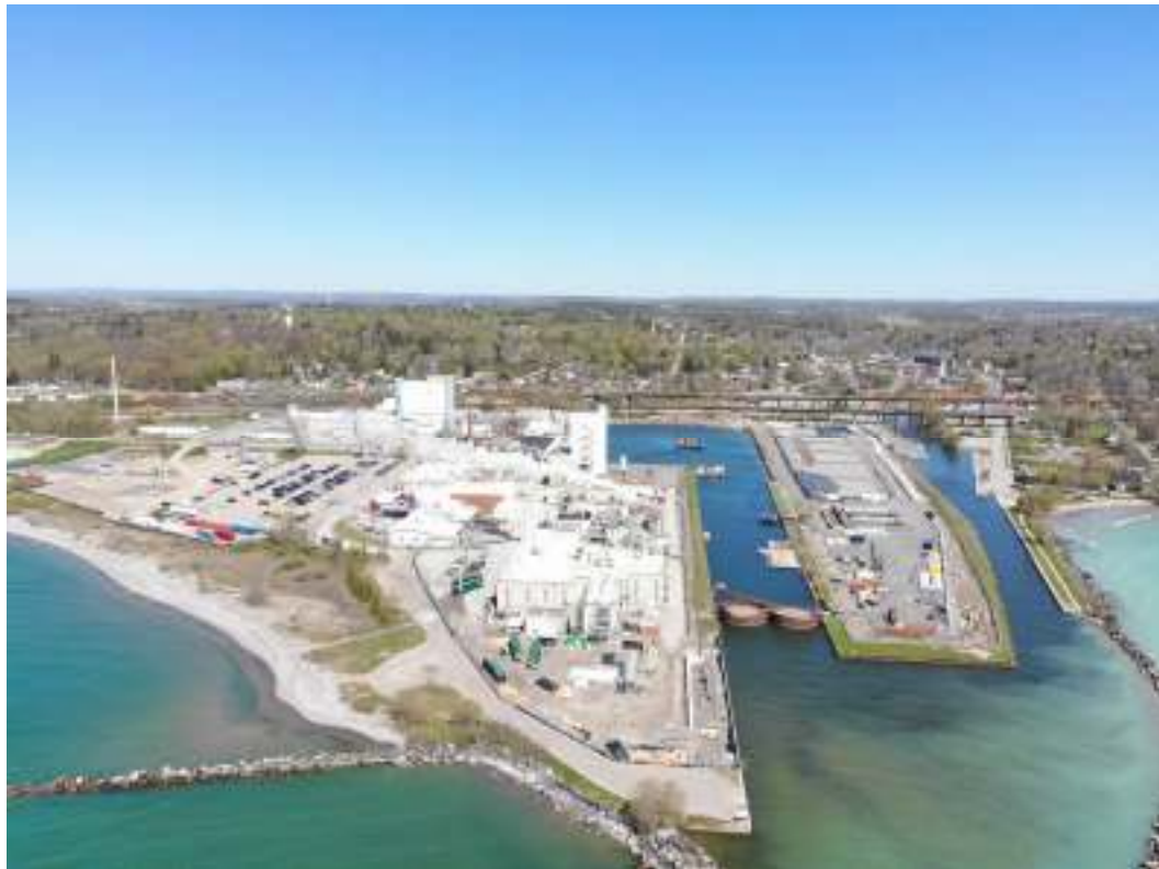
Figure 1 – Site 1 - Port Hope Conversion Facility
