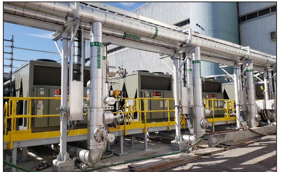
Components of the new closed loop cooling system at the Port Hope Conversion Facility. Lake water is no longer used to cool production process at the facility.
