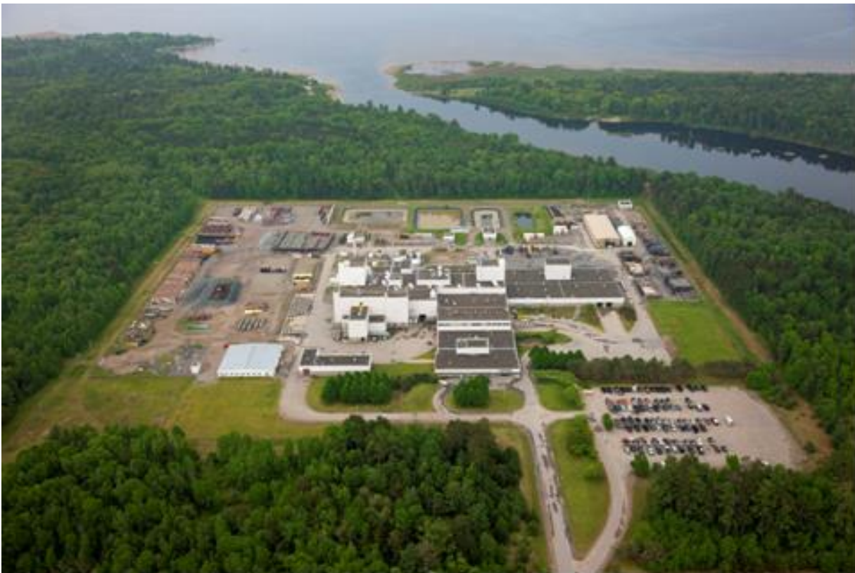
Figure 1 Blind River Refinery
